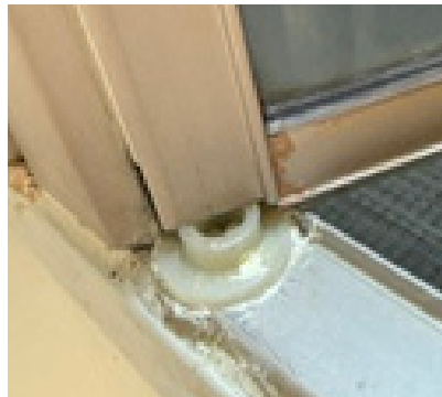
Washer epoxied into place
